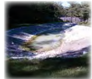
PondSeal was used by Crystal Springs Trout Farm (MI) to seal this pond
