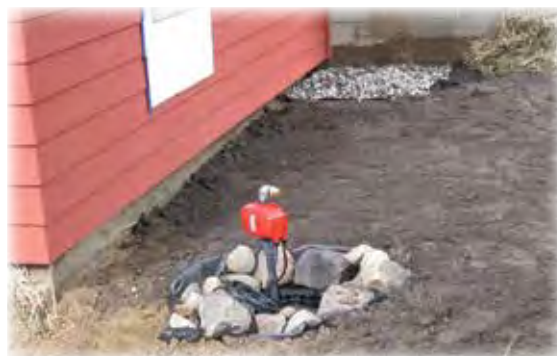
A 1000 gallon system was installed under a future patio area in this backyard setting. The 6' x 11' reservoir area was reduced to only a 24" diameter visible area.
