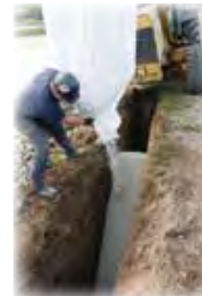
Great for sealing earthen dams and dikes!
